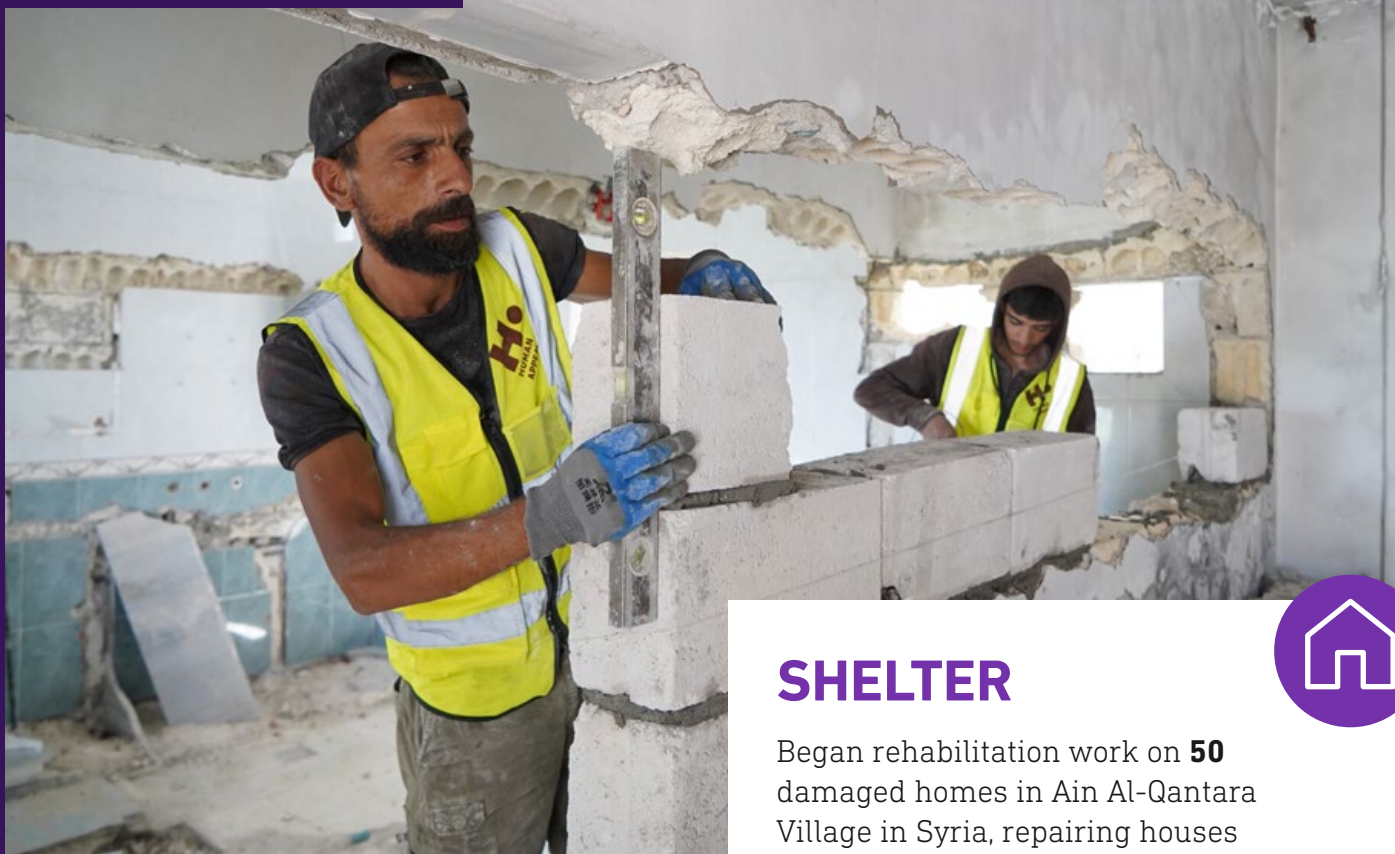
Rehabilitating the damaged walls of a house.
