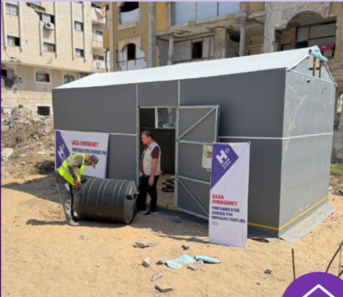
Setting up one of the shelters.
