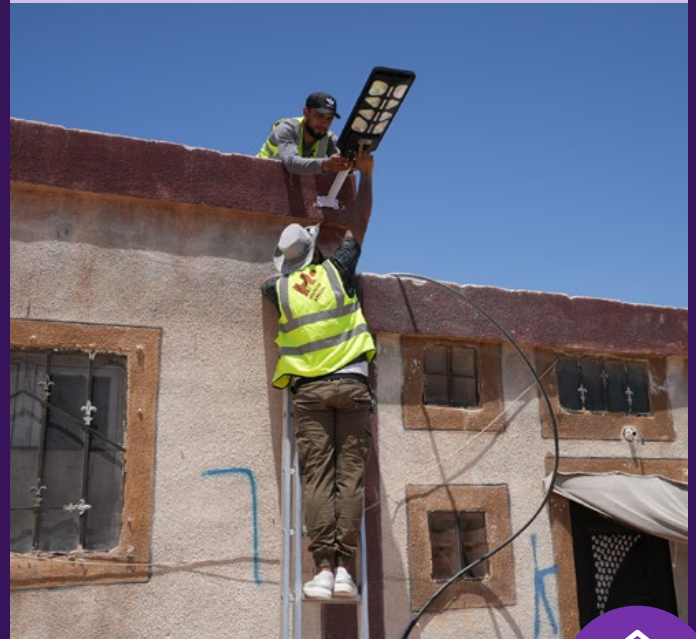
Installation of the street lamps in progress.
