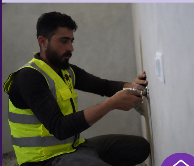
Rehabilitation of home in progress.
